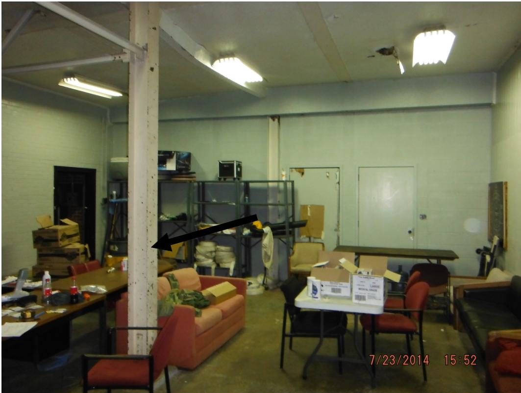
Lead-based paint on structural column and angle-iron bracing in supply area #5
