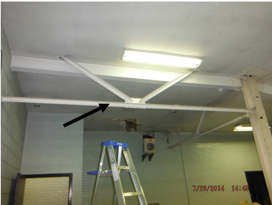
Lead-based paint on structural column and angle-iron bracing in supply area #5
