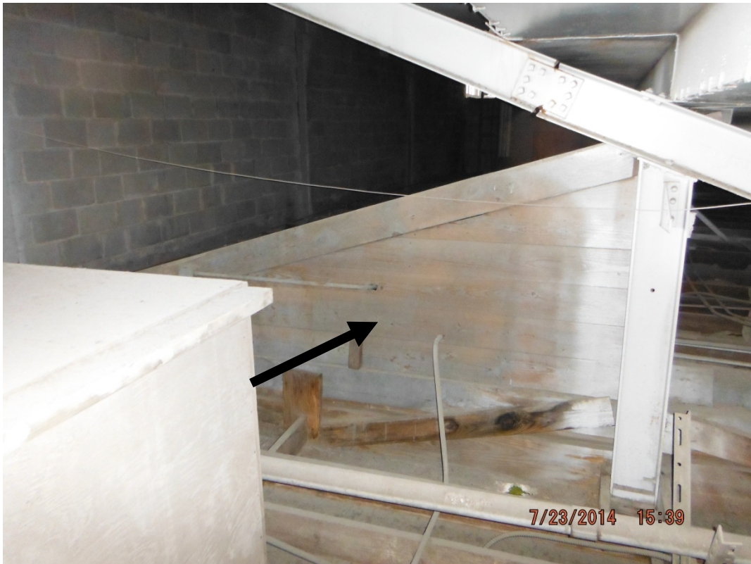
Lead-based paint on wooden wall from previous structure on top of existing structure
