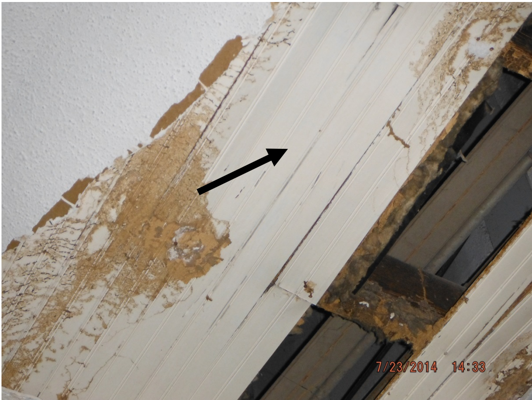
Lead-based paint on tongue-n-groove ceiling above the textured drywall ceiling in supply area #5
