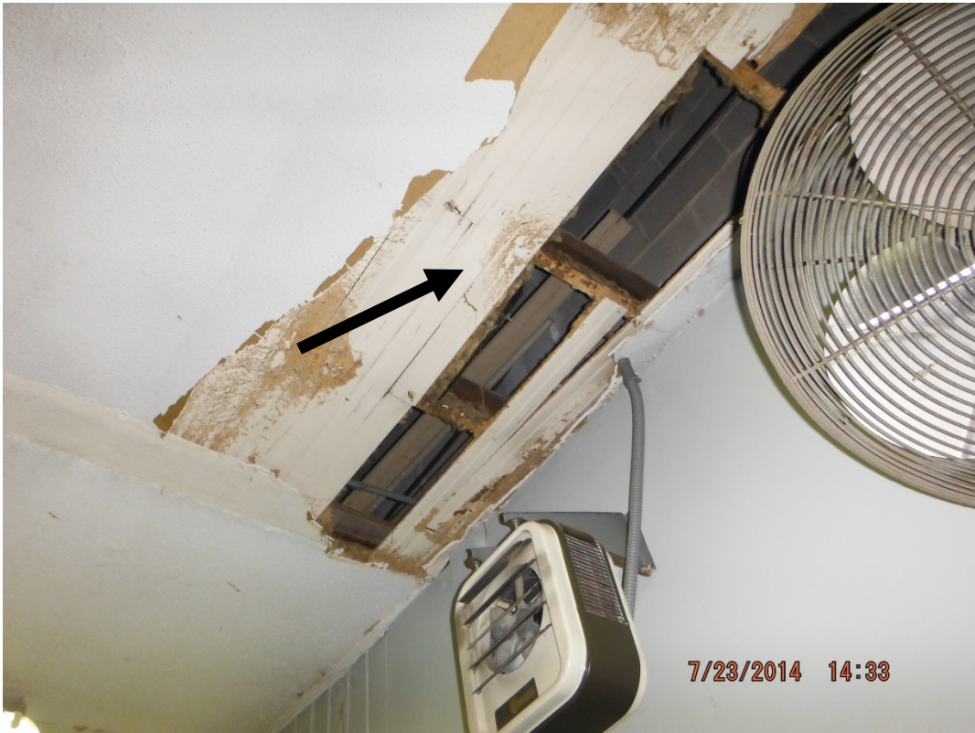
Lead-based paint on tongue-n-groove ceiling above the textured drywall ceiling in supply area #5
