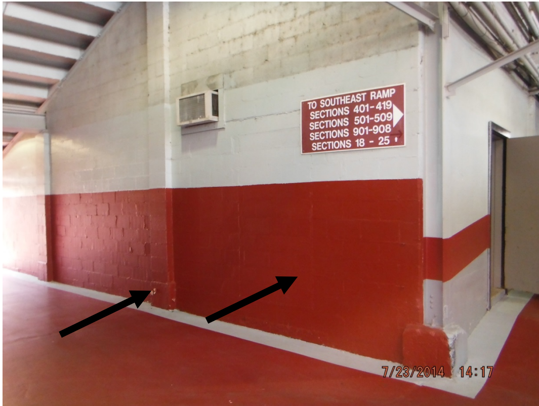
Lead-based paint on maroon painted wall and columns on south end exterior wall; may be an underlying paint that contains the lead
