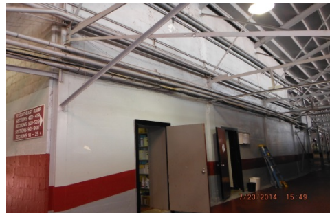
Photo 1. Exterior of the subject structure includes concrete, masonry block and brick walls.
