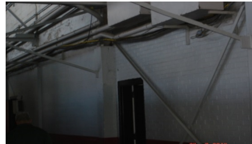
Photo 1. Exterior of the subject structure includes concrete, masonry block and brick walls.
