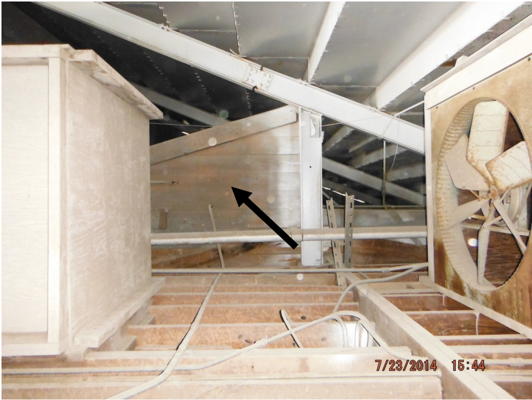
Lead-based paint on wooden wall from previous structure on top of existing structure
